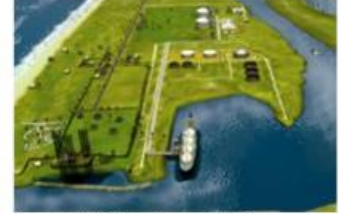
*Freeport LNG Development, L.P. Cheniere Energy, Inc. 30%
