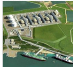
SPA with CCL First LNG Expected 2018
