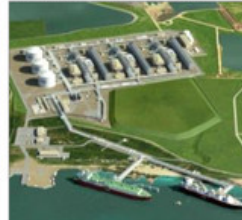
SPAs with CCL First LNG Expected 2018
