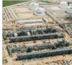
SPA with SPL First LNG for SPL Expected 2015
