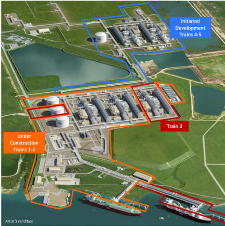
Design production capacity is expected to be ~4.5 mtpa per train, using ConocoPhillips' Optimized Cascade® Process
