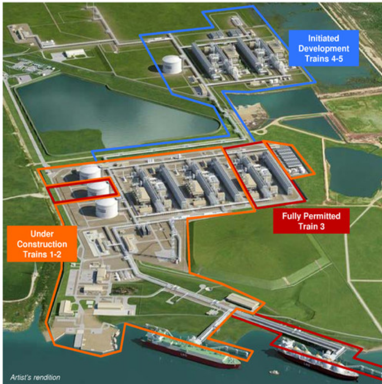
Artist's rendition Adjusted nominal capacity is expected to be 4.3-4.6 mtpa per train, using ConocoPhillips' Optimized Cascade® Process. Please see the appendix for more detail on the adjusted nominal capacity.
